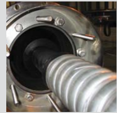
STRESS CONE POSITIONING
