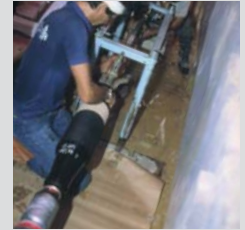
Joint sleeve positioning
