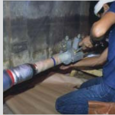
Cable head preparation
