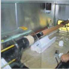
Joint sleeve expansion on carrier tube
