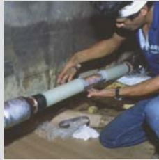
Corona shield positioning
