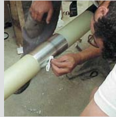
Cable core finishing
