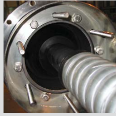
STRESS CONE POSITIONING
