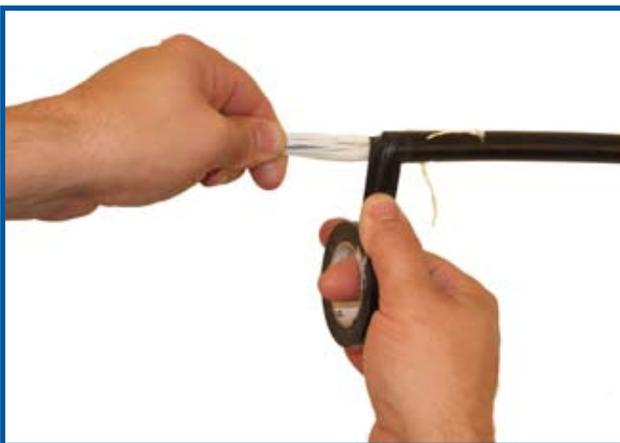
7. Slide the pulling grip back up over the cable end so that the cable core extends about 1/4 to 1/2" beyond the weave section of the grip.
