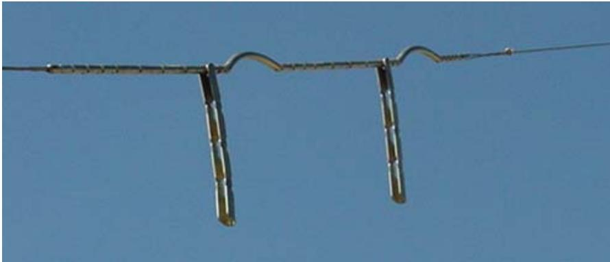
Fig 6. Anti-twisting devices
